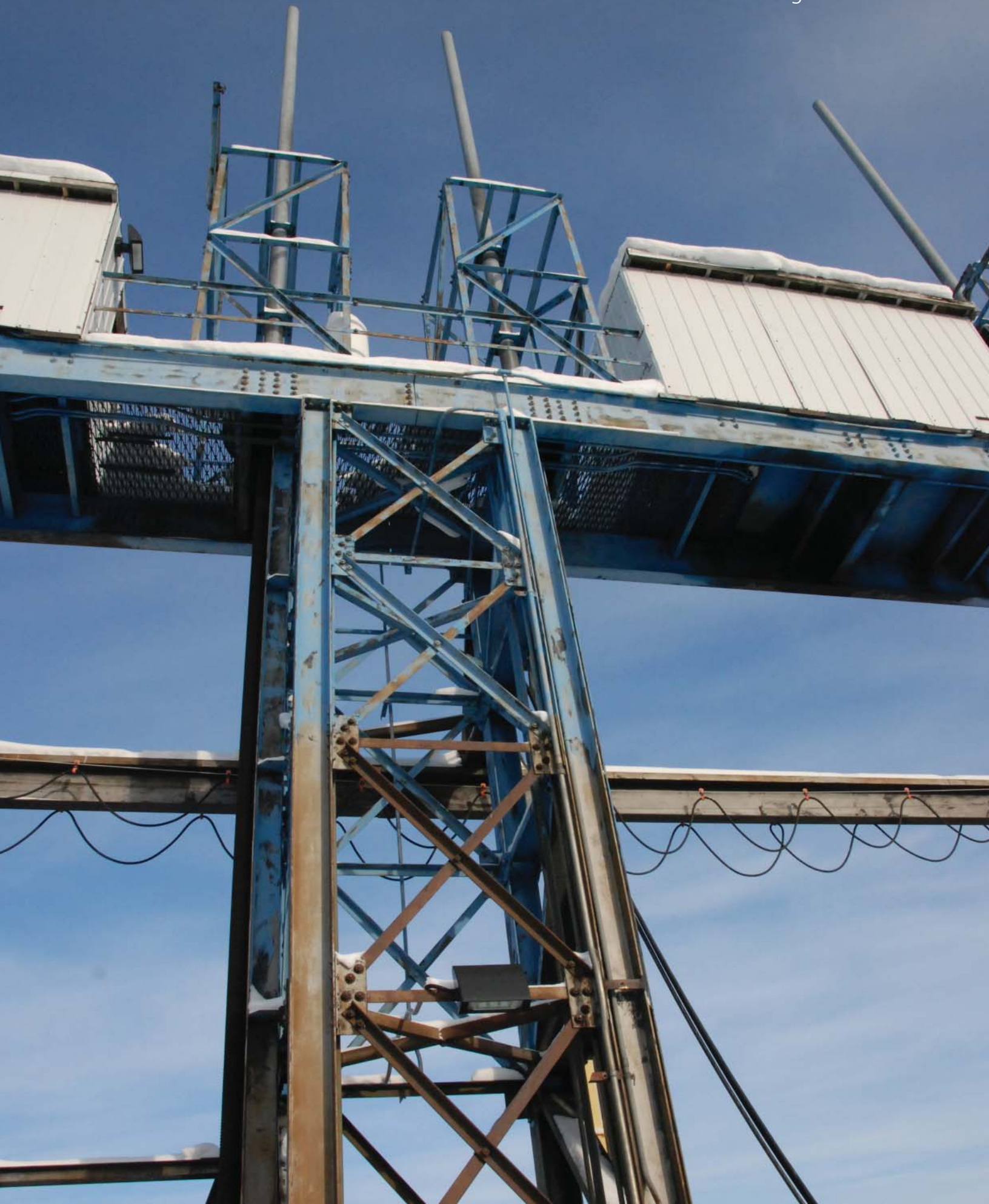
Snare Falls headgate structure.
