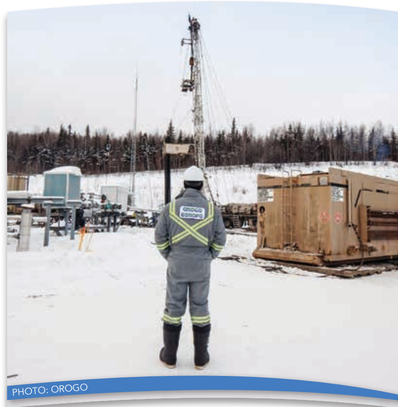
Mischa Malakoe (Safety Officer) inspecting a well abandonment in the South Liard Field, March 2017.
