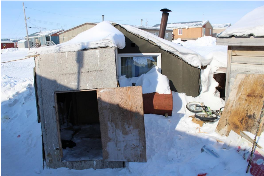
Due to the severe housing shortage, a young family in Igloolik, Nunavut lived in this poorly constructed wooden shed.
