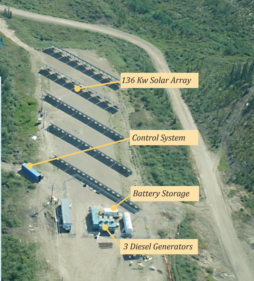
Aerial of Colville Lake Pilot Project
