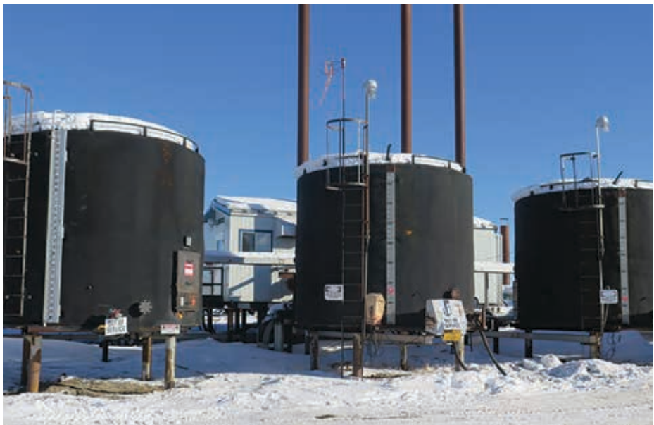
Fuel and chemical tanks cleaned out and tagged as out of service, Cameron Hills, March 2019. (Credit: GNWT Lands)
