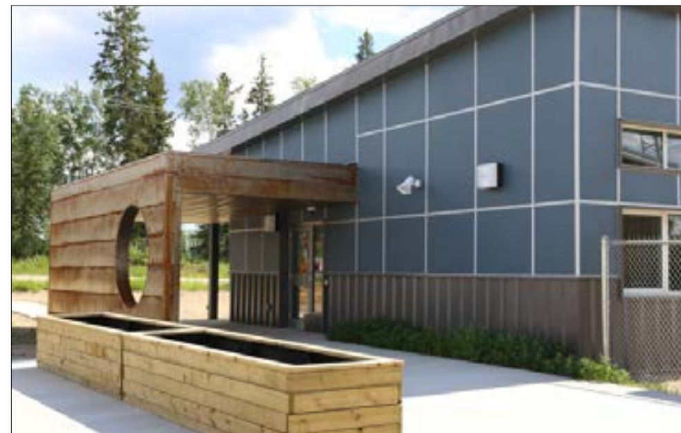
The Centre for Mine and Industry Training was completed in the summer of 2018 for occupancy in September. The facility will house the majority of mine-related training, as well as educational equipment such as simulators and vehicles.
