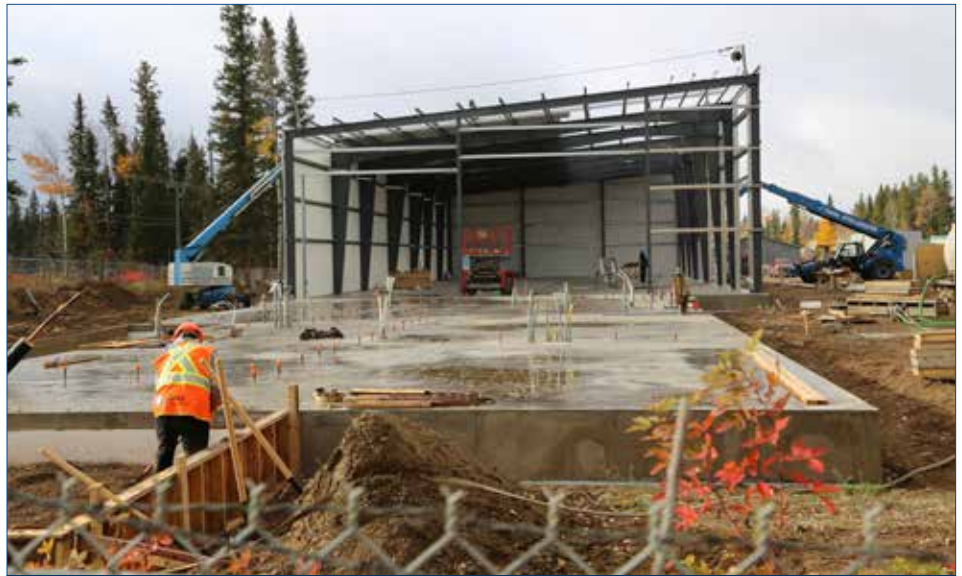
The Centre for Mine & Industry Training will be completed by March 31, 2018.
