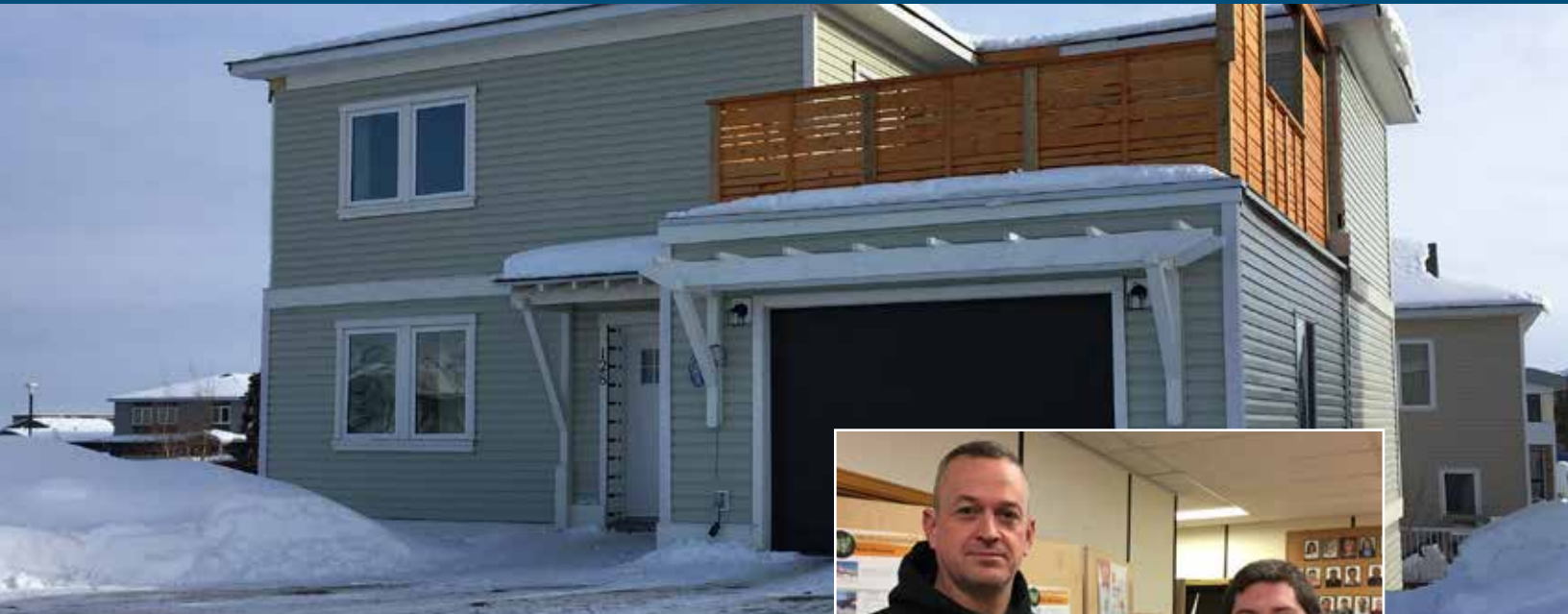
Michael Goodwin of the AEA presents David LeBlanc with a rebate cheque for building a home with an energy-efficiency score of at least 85 out of 100.
