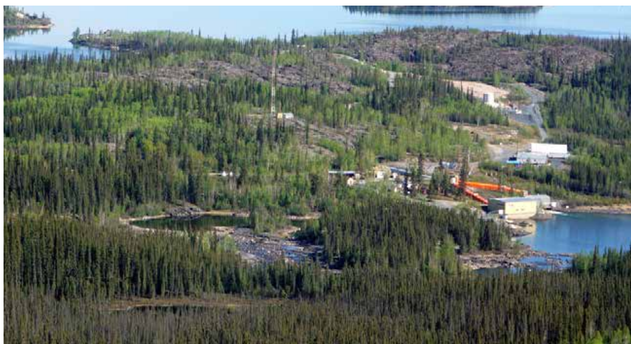
Aerial view of the Bluefish Generating Station
