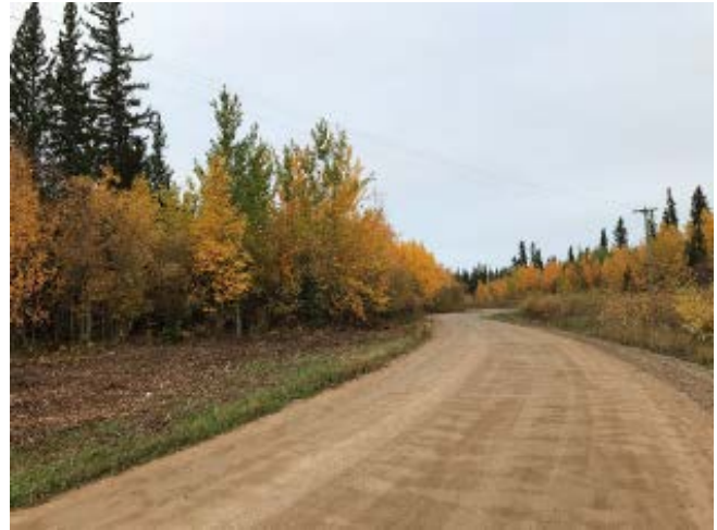
A bend in the Hay River Beach Access Road .
