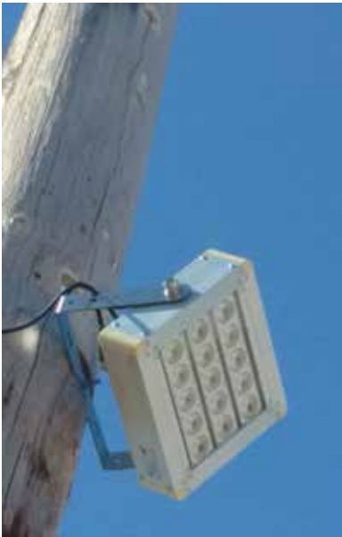
New LED Light Fixture.
