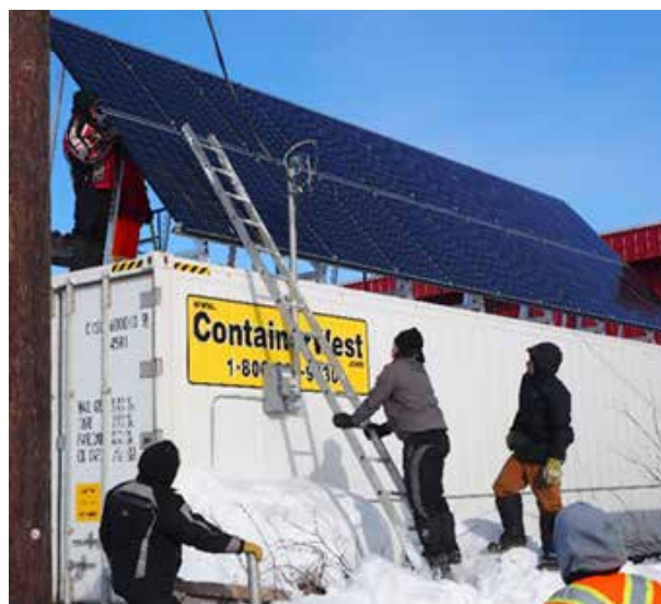
Installing solar panels on the Community Freezer in Inuvik.
