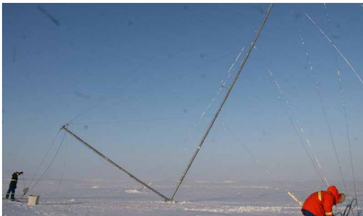
Installation of Beaufort Wind Monitoring Tower.
