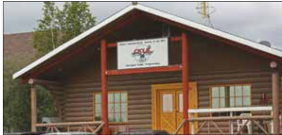
CKLB 101.9 Radio building in Yellowknife.
