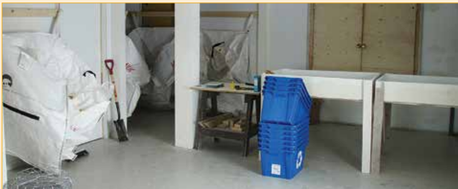
The renovated interior of the Ulukhaktok recycling depot.
