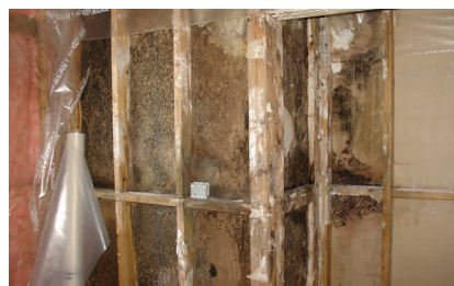
Maurice St. Martin's Home During the Renovations
