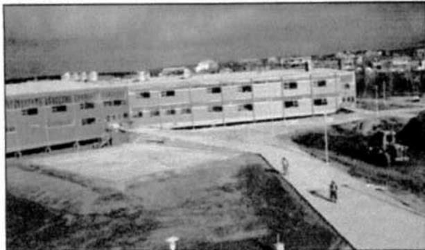
A view of the back of the mega construction project.
