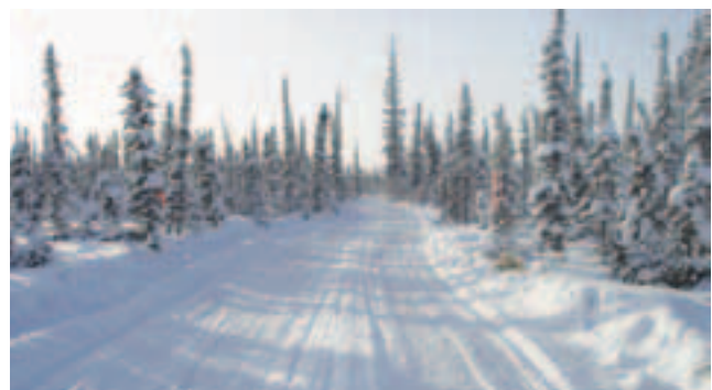
FIGURE 26. (LEFT) Leaners on this recently cleared seismic line should be removed and more snow or ice is required to protect the ground surface. (RIGHT) An acceptable seismic line with no leaners and adequate packed snow.
