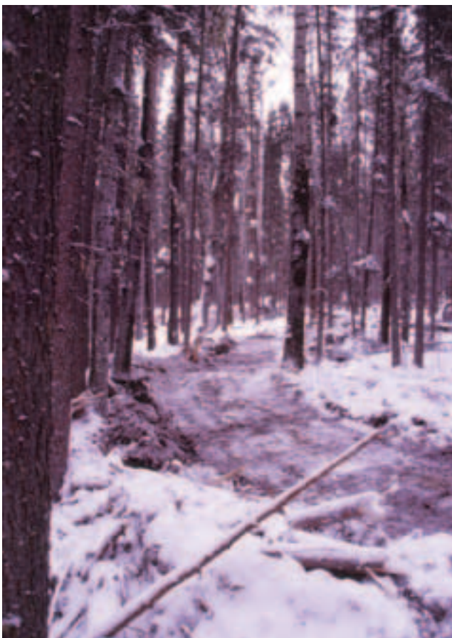
FIGURE 15. A good example of a meandering line cut to avoid large trees; however, there is insufficient snow on the ground to prevent surface disturbance.
