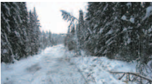
FIGURE 26. (LEFT) Leaners on this recently cleared seismic line should be removed and more snow or ice is required to protect the ground surface. (RIGHT) An acceptable seismic line with no leaners and adequate packed snow.
