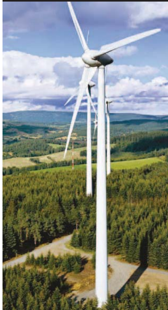
Figure 14: A Wind Farm - Source: Environment Canada
