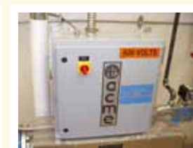
Highways Maintenance Garage Boiler Type:..... Acme Size:.....83 kW
