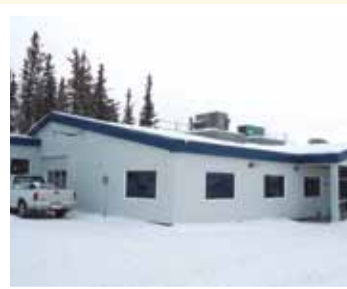
Energy Upgrades - Ventilation North Slave Regional Office (PWS), Yellowknife
