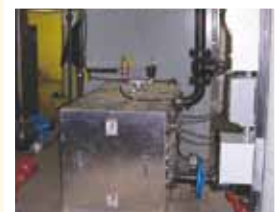
Breynat Hall Boiler Type: .....Acme Size: .....720 kW
