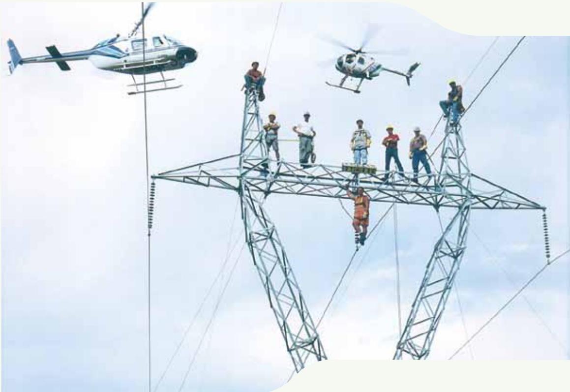
Constructing a transmission line in the NWT.
