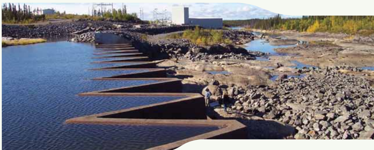
The Snare Cascades spillway.
