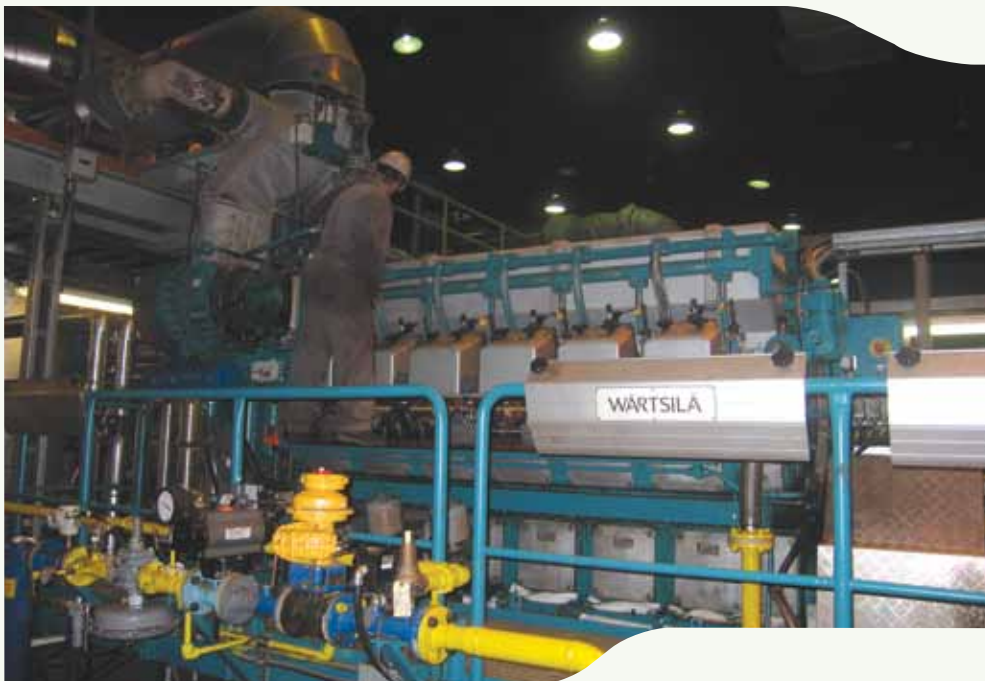
Natural gas turbines at the Inuvik generation plant.
