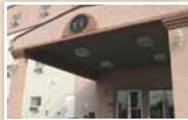
CHATEAU NOVA HOTEL AND SUITES www.chateaunova.com 80 rooms including suites
