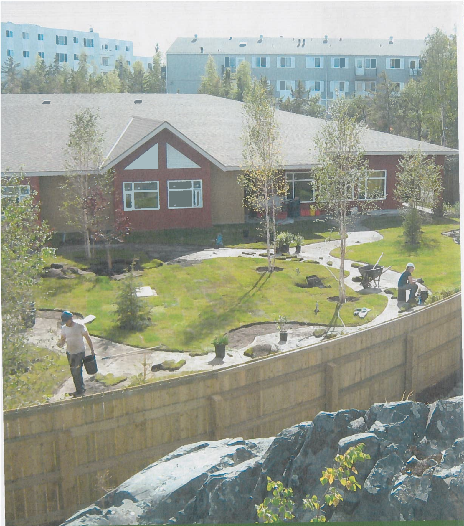
A look into the courtyard of the new Territorial Dementia Facility. PWS photo
