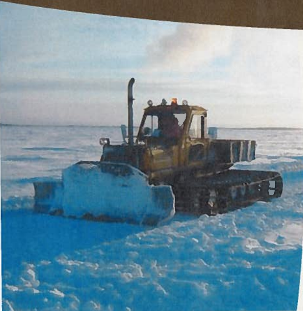
A plow puts the finishing touches to the ice road on Marion Lake. DOT photo
