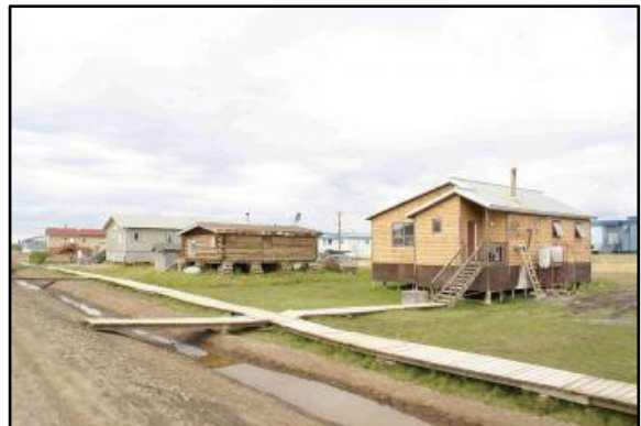
Photo 3.1.1 Aklavik roads, sidewalks & houses
