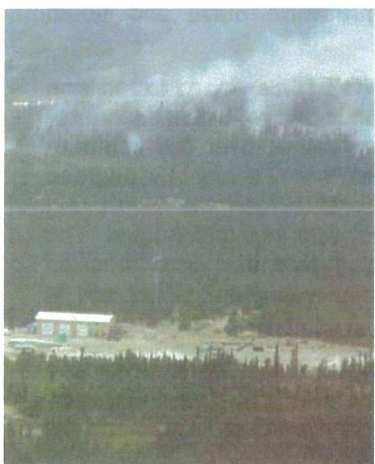
Snare Lake Hydro Complex (ZF-030-08)
