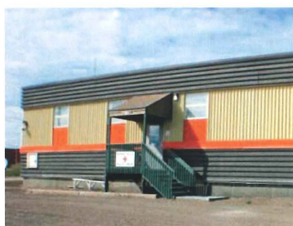
Norman Wells Health Centre
