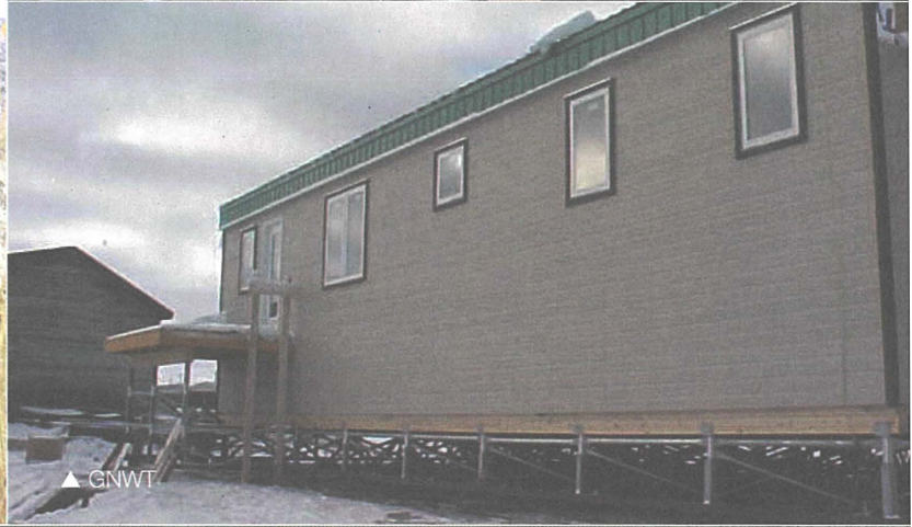
▲ Foundations that distribute weight and absorb stress limit problems caused by ground movement – Tridetic Building Products Ltd.
