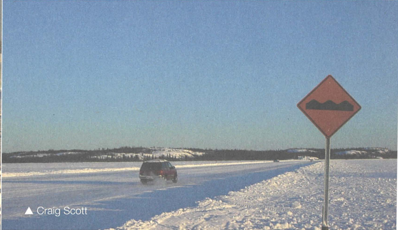
▲ Bridges on Mackenzie Valley winter road – GNWT
