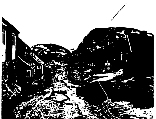
General layout of streets and homes in Sukkertoppen. This is a problem in rocky areas.
