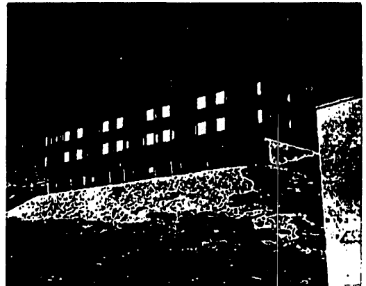
Beautiful design apartment for Greenland Air pilots in Godthaab. Cost per square metre to build is the same as the pre-cast concrete construction. These units have more floor space and superior quality.
