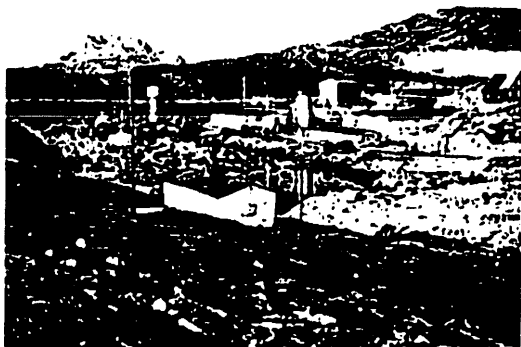
Godthaab harbour. Whole hills of rock is blasted away to make a landing site and area for fish plant.
