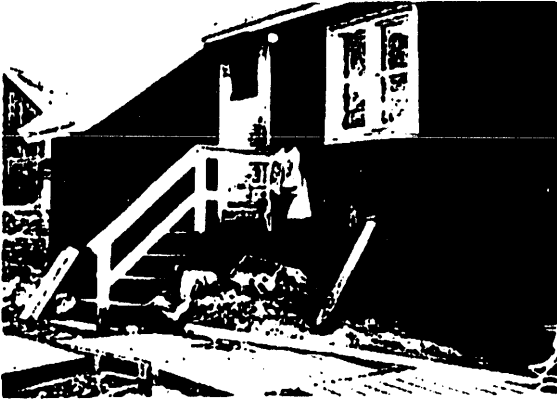
Kitchen water is drained out in front of the home, garbage is a problem during winter. Note the bags hanging out near the front door. Meat is left out to cool.
