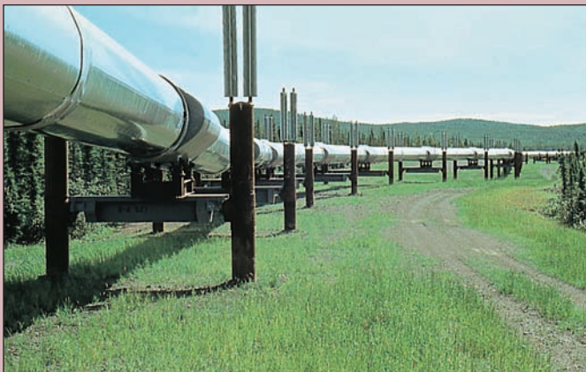
Pillars hold up sections of the Trans-Alaska Pipeline so that it will not be affected by permafrost.
