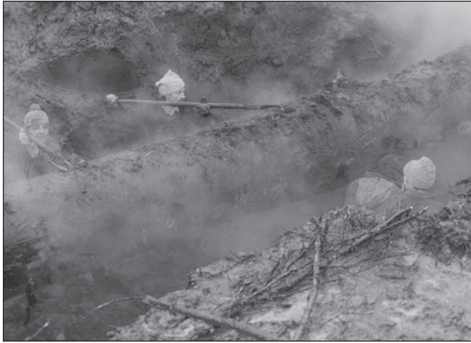
Workers look for a leak on an old oil pipeline near Usinsk, Russia in 1994. They were trying to stop an oil spill that had polluted two rivers near the Arctic Circle.
