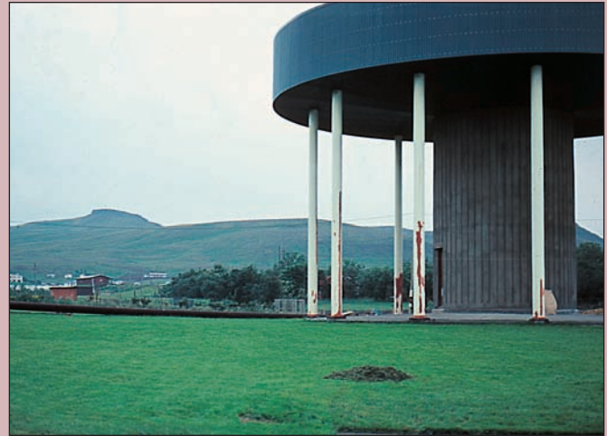
This tower holds hot water from thermal springs. From this tower, the water can be piped to buildings. The average natural temperature of the water is 80°C.
