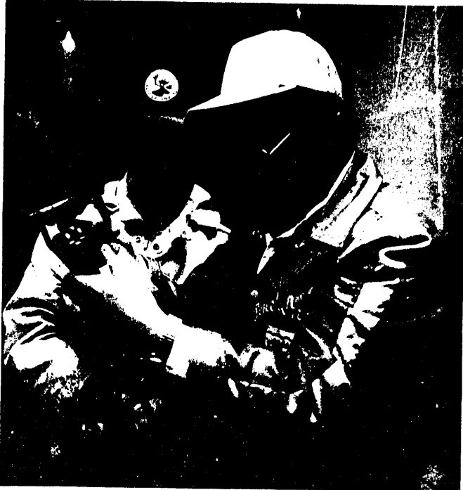
DPW supervisor Joe Koonoo and assistant Pauloo Sangoya check the school boilers in Pond Inlet.
