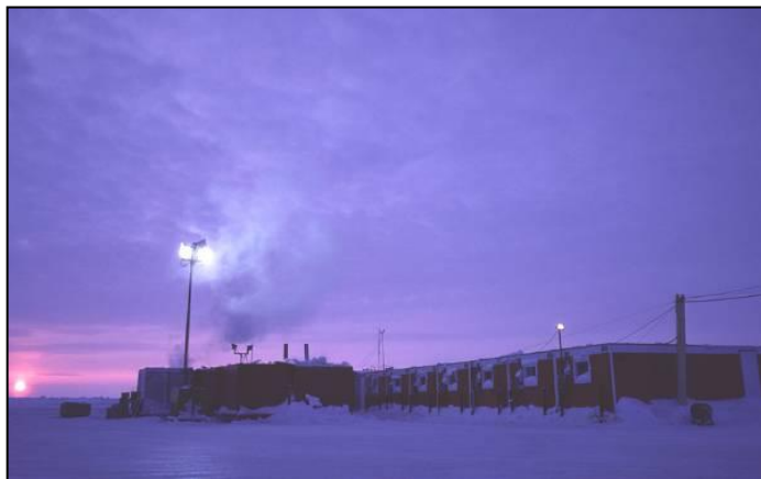
Smoke stack in the Arctic (Photo: stock photo)
