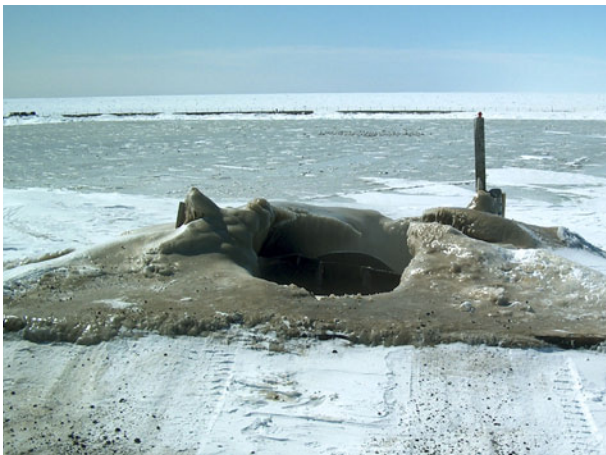
Sewage disposal site , Arviat, Nunavut
