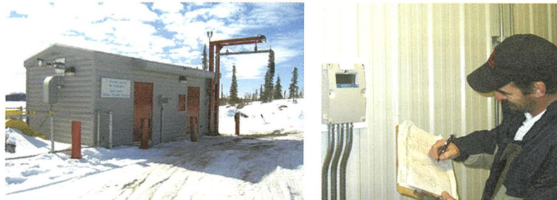
Picture on the left: Small System WTP in Gamètì.
