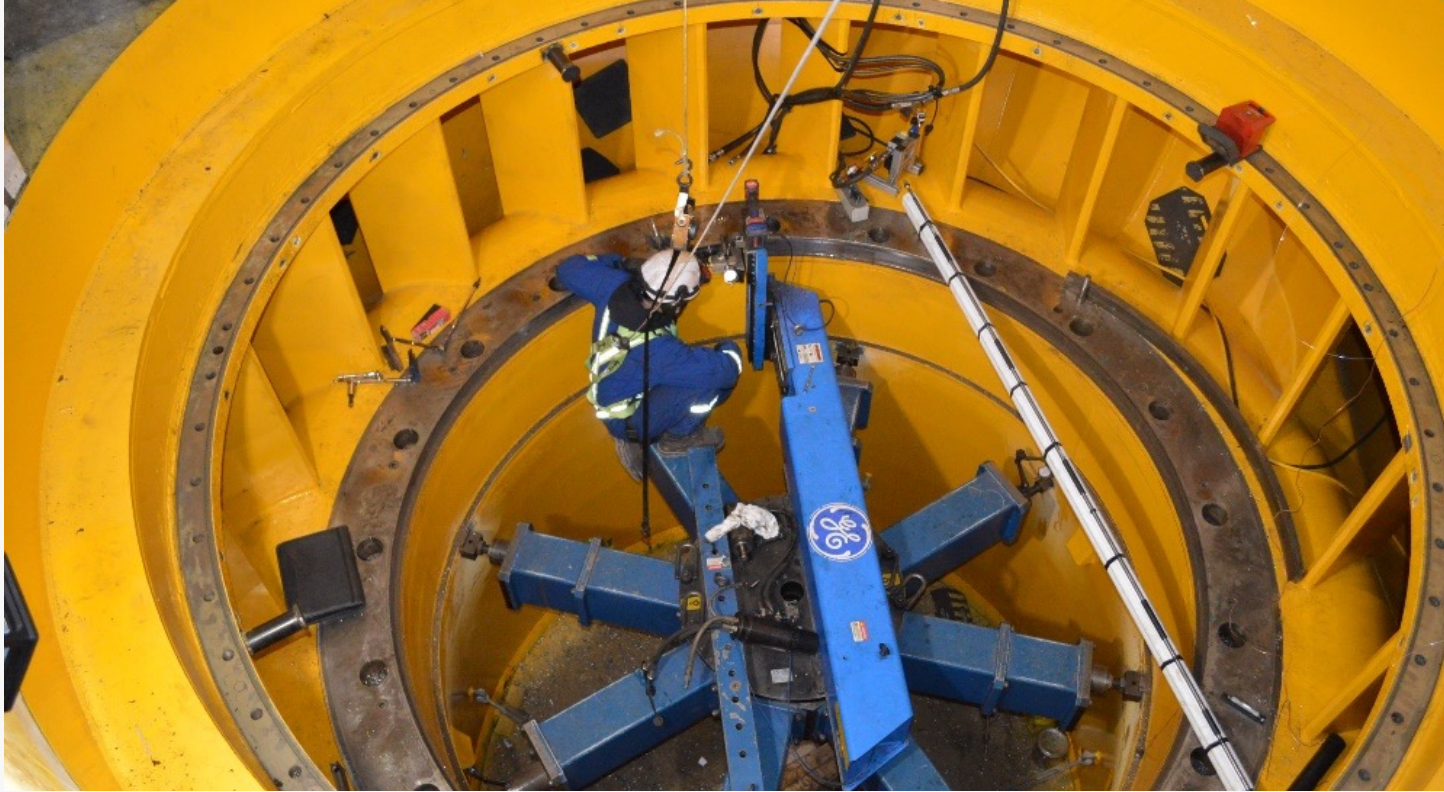
Work on refurbishment of Snare Forks Unit 1 continued in 2020-21
