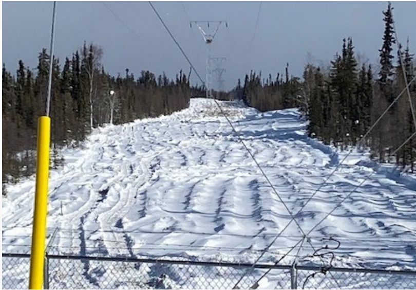
Keeping vegetation away from transmission and distribution lines helps to reduce the frequency of outages
