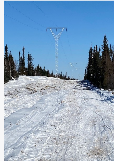
Keeping vegetation away from transmission and distribution lines helps to reduce the frequency of outages
