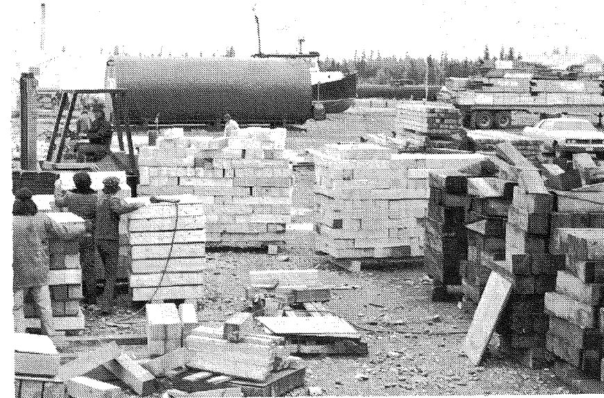
Prefabrication activities in Hay River
