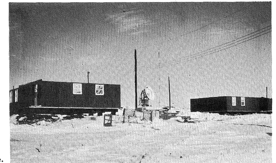
Erection of typical prefabricated house package.
