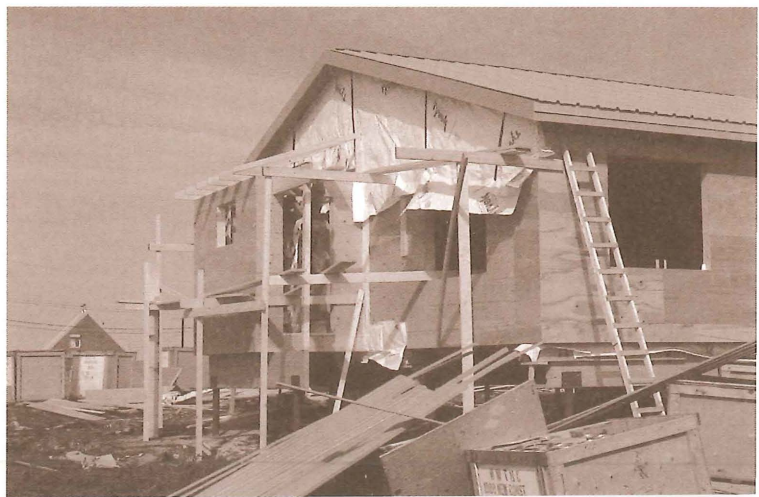
Exterior of a housing unit nearing completion.
