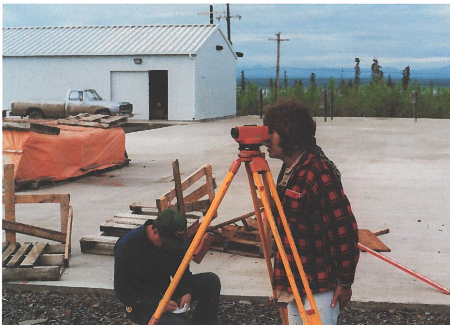
Survey Team Laying Out Air Tanker Base - Norman Wells
