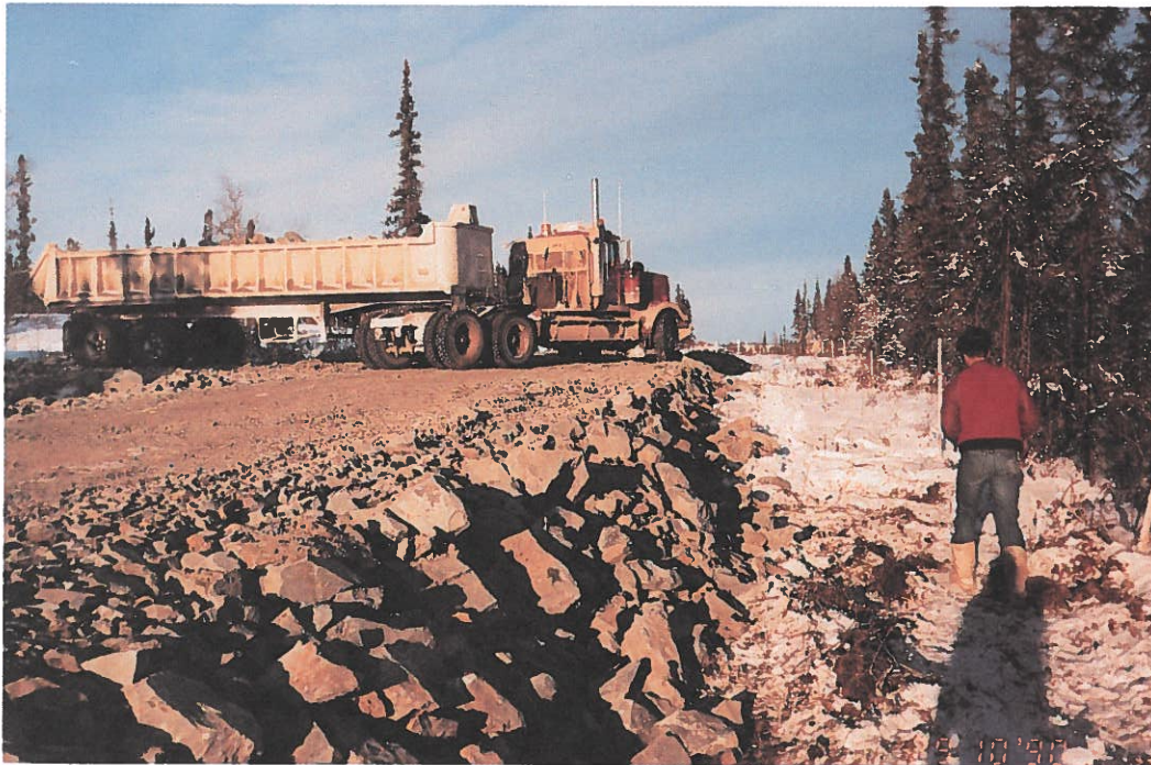
Construction of Road to Sewage Lagoon - Dettah
