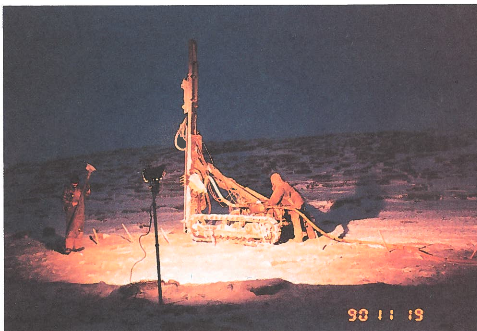
Night Drilling - Repulse Bay
