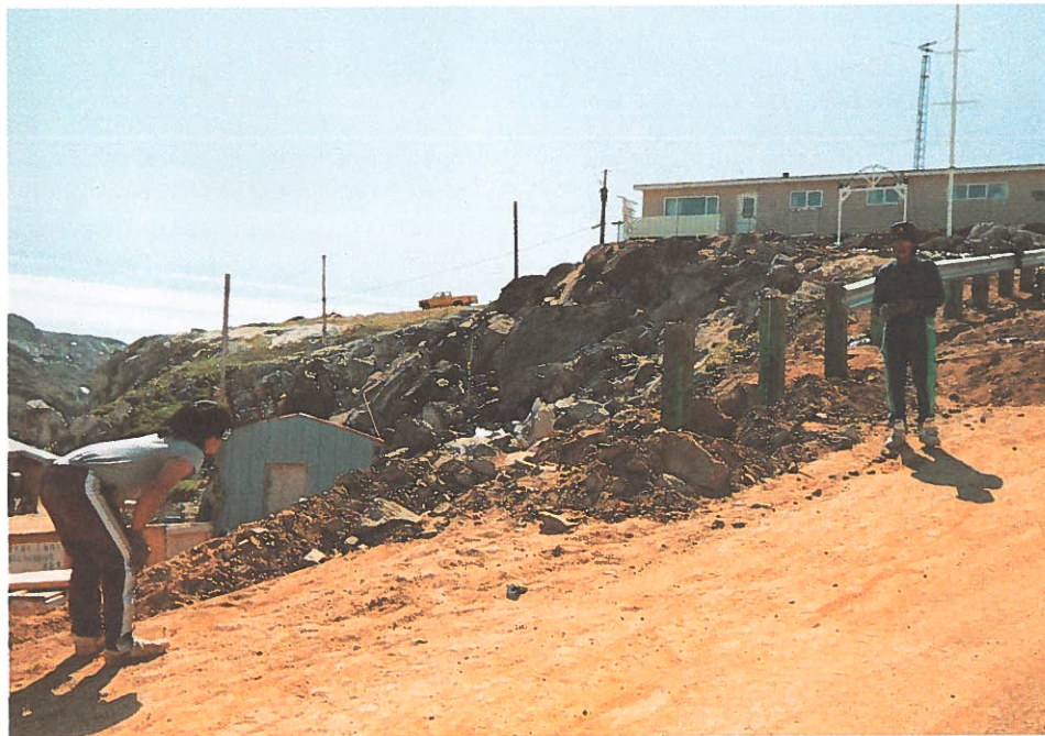
Local Work Force Installing Guard Rail - Lake Harbour
