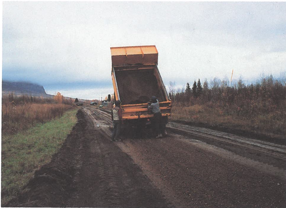
Spreading Surfacing Gravel on Sewage Lagoon Road - Nahanni Butte
