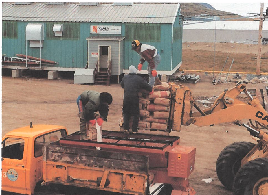
Filling Spreader Hopper with Calcium Chloride - Pangnirtung
