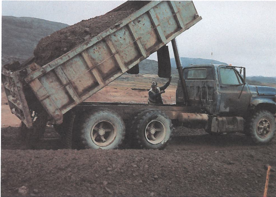
Truck Dumping Gravel for Road Construction - Cape Dorset
