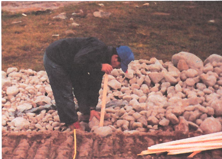
Survey Assistant Setting Slope Stakes - Pangnirtung
