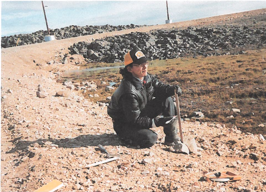
Survey Assistant Placing Shoulder Stakes - Cape Dorset
