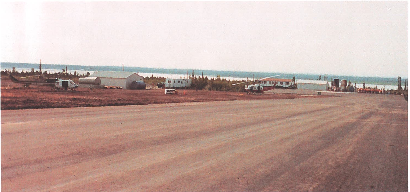
Air Tanker Base and Heliport Construction - Norman Wells
