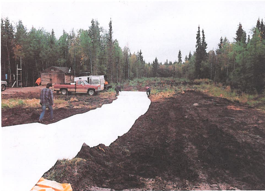
Laying Geotextile on Sub-grade - Hay River Reserve
