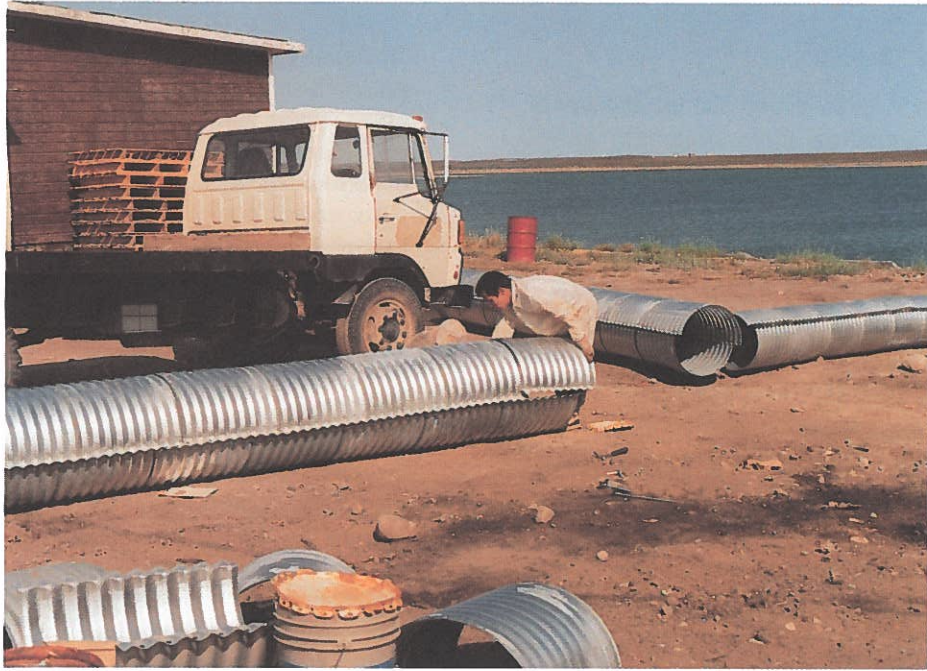
Assembling Nestable Culvert for Drainage Improvements - Arviat
