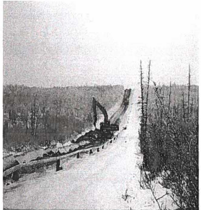
Constructing the Ikhil Gas Pipeline
