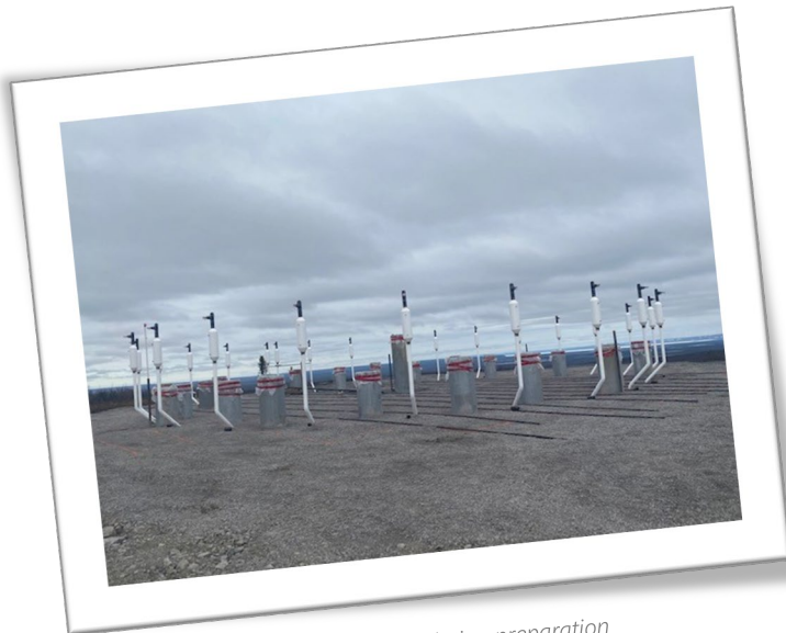
Inuvik High Point Wind Project foundation preparation
