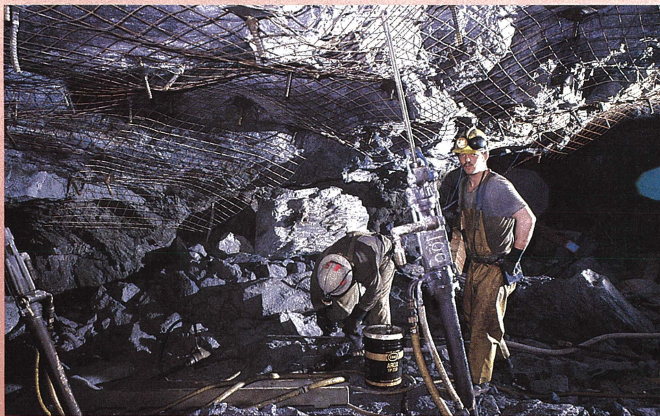
4. Underground crew at the Nerco mine in Yellowknife installing wall support.
