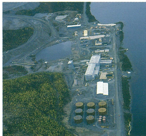
Colomac gold mine at Baton Lake officially started operations in late August.
