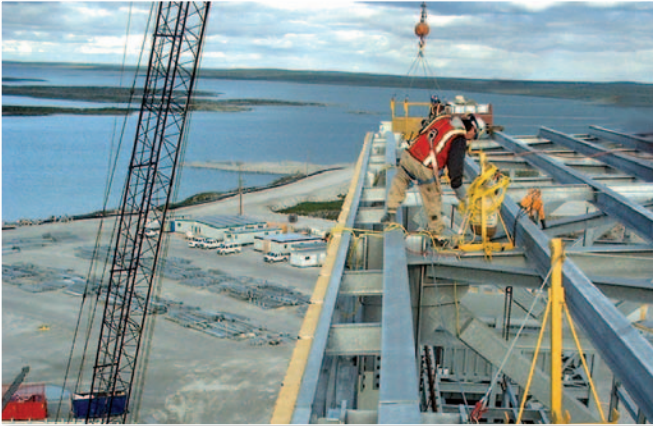
Construction at Diavik Diamond Mine (Photo: Diavik)
