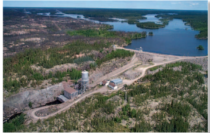
Taltson Hydroelectric Facility (Photo: NTPC)
