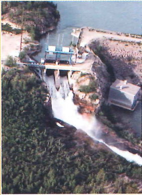
Located 15 km southwest of Snare Rapids, the Johnny Simpson Power Plant is the second downstream hydro plant on the Snare River. Commissioned in 1961, the plant can generate 7.5 MW from a variable pitch turbine.
