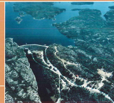
Aerial photo of the Ted Humphry's Plant at Snare Rapids.
