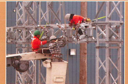
25kv Upgrade of Inuvik Substation - Summer 2005
