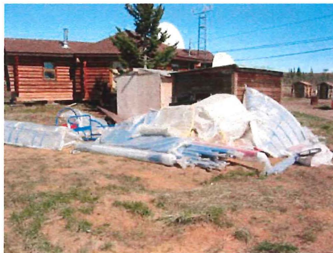
Equipment arrives to begin construction of a playground in Colville Lake.
