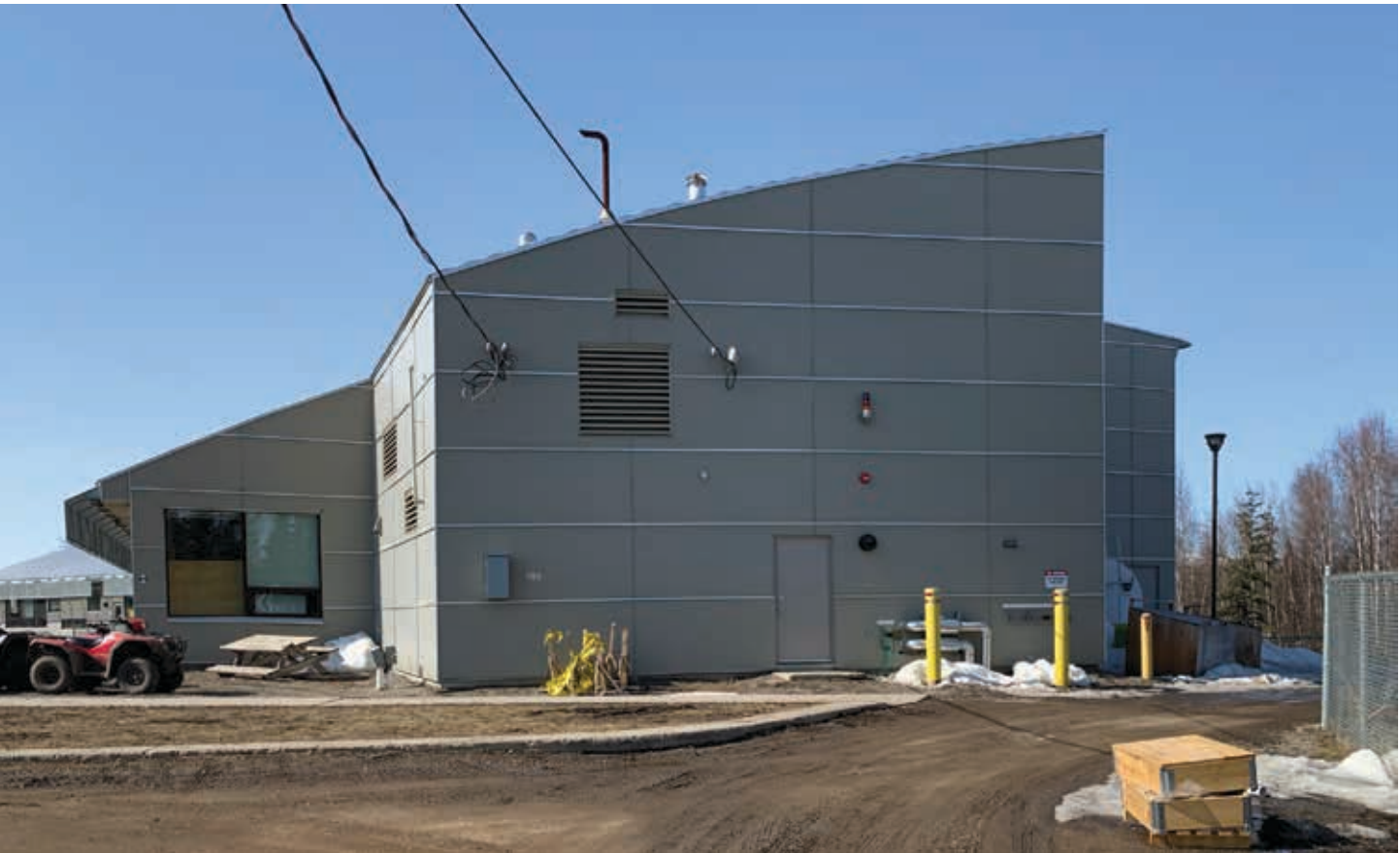
Tulita's Chief Albert Wright School has been switched to more energy efficient LED lighting.
