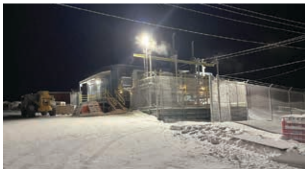
Construction continues on the new Sachs Harbour power plant.
