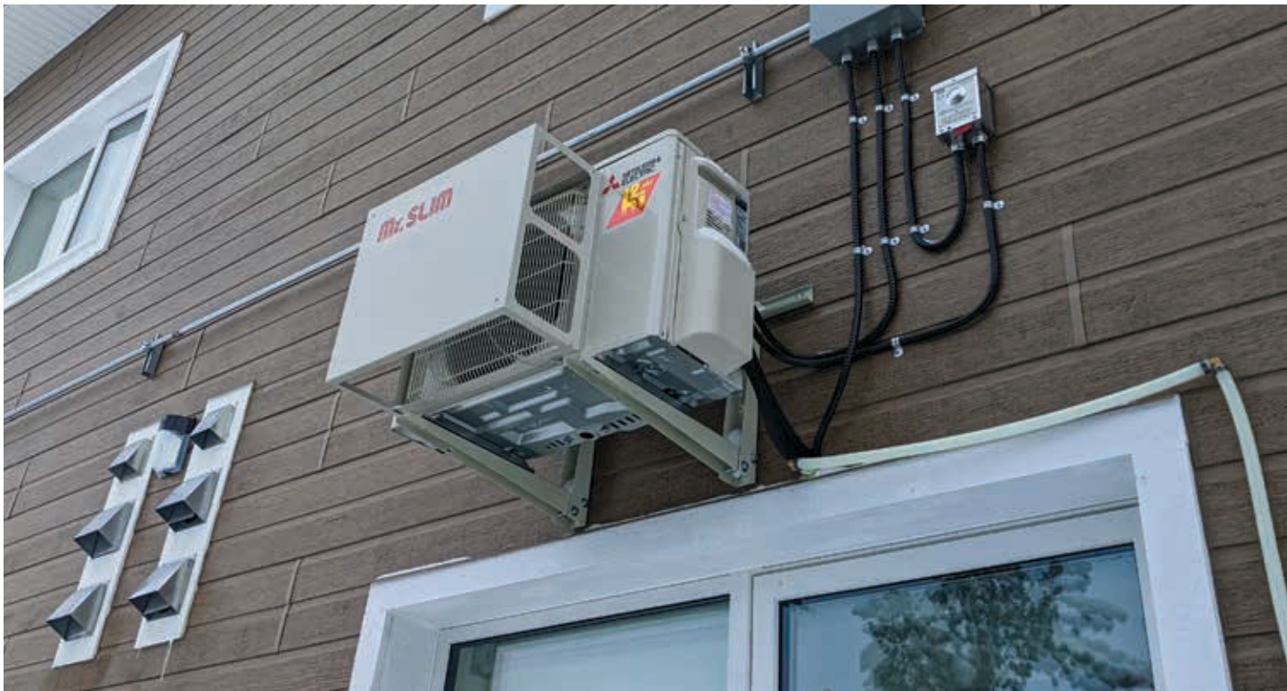
The AEA has started a project to see if cold-climate heat pumps could work in the NWT.
