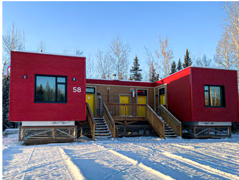
New modular fourplex in Nahanni Butte, NWT Photo Credit: Housing NWT
