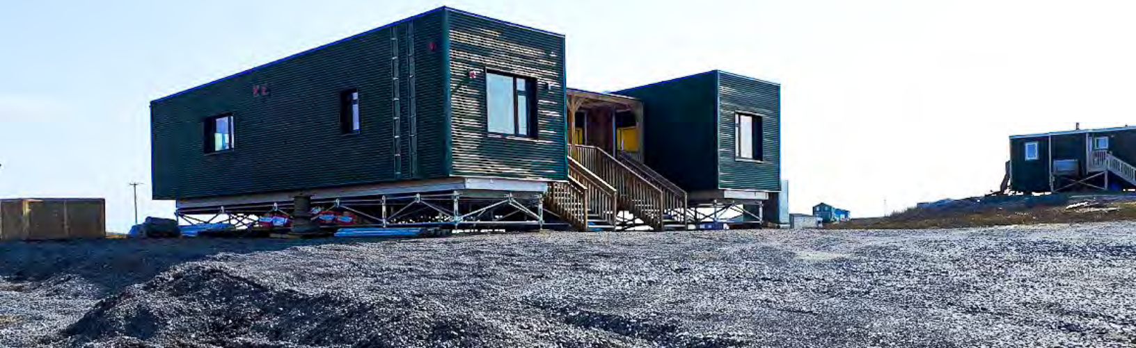
New modular fourplex in Tuktoyaktuk, NWT Photo Credit: Housing NWT
