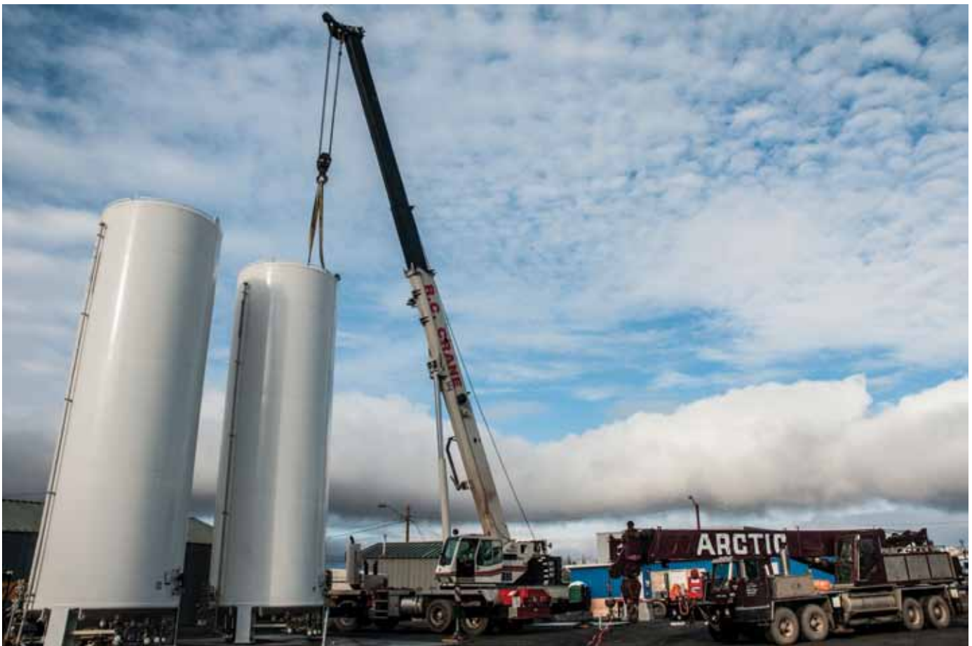
Installation of Northwest Territories Power Corporation's LNG tanks in Inuvik.
