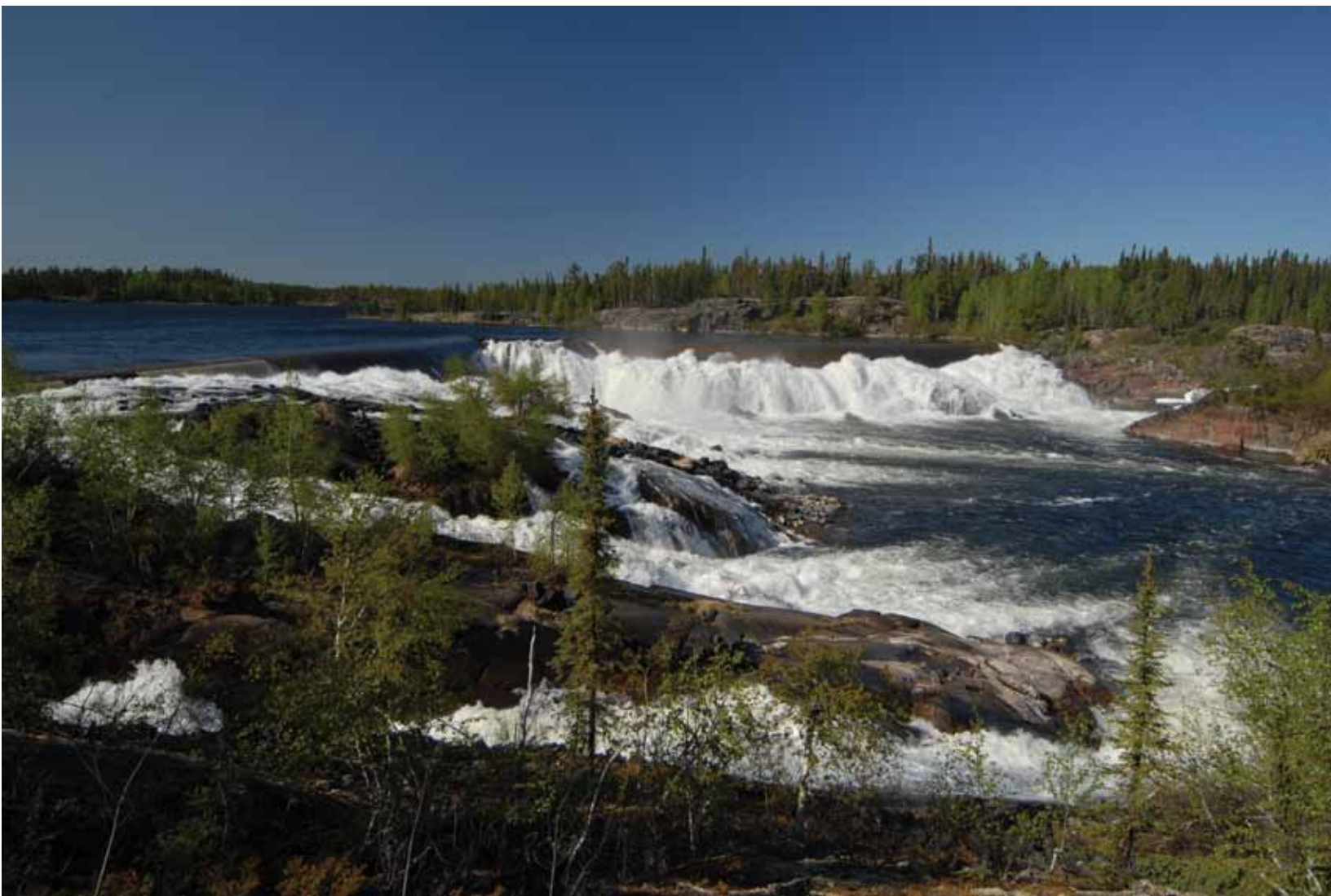
South Valley Spillway, Taltson River
