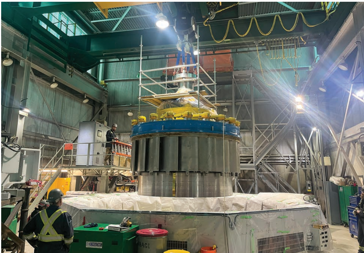
Generator being installed
