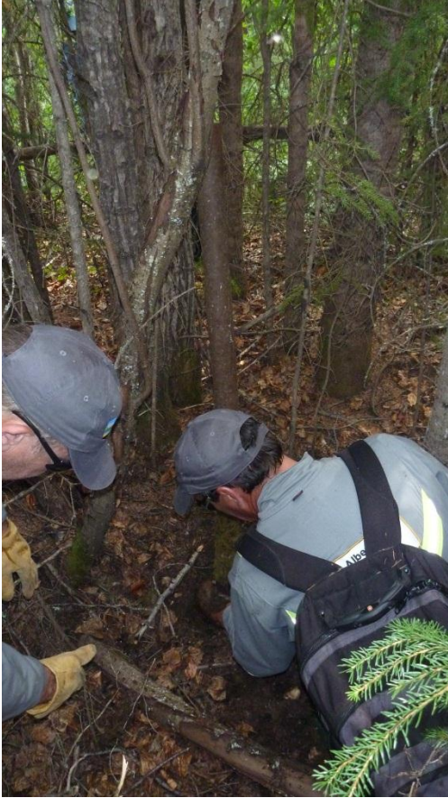
JMR No. 1 Well: Uncovering wellhead and cap
