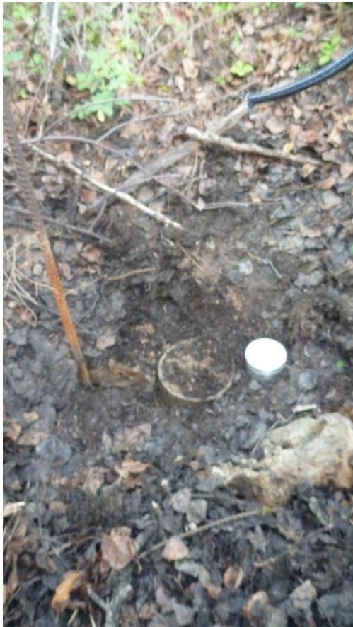
Westerol 3A Well: Wellhead with soil detector cap
